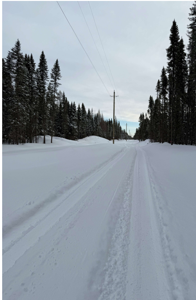
Hydro Line energized
