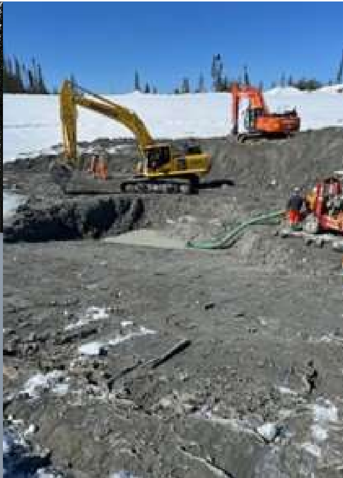
Box cut to bedrock
