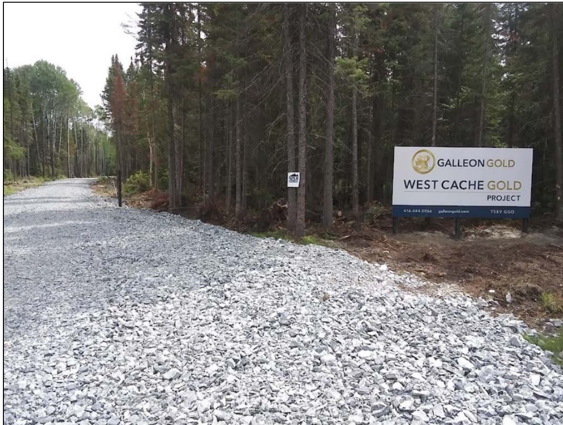
FIGURE 5.2 ACCESS ROAD AT PROJECT ENTRANCE OFF HIGHWAY 101
